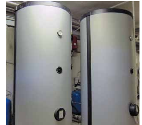
New hot water tanks
