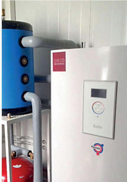
Thermia Solid ground source heat pump
