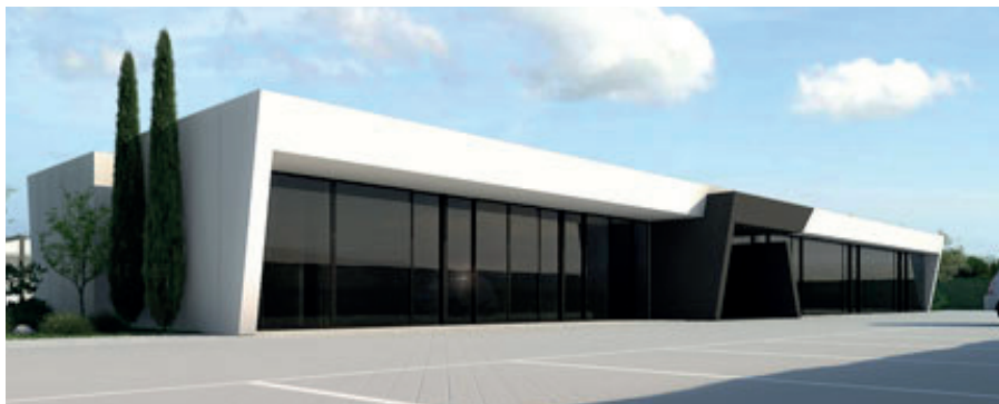
Exterior view from the courtyard
