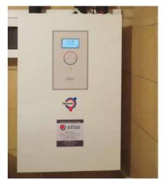
is set at 30°C when the outdoor temperature is at + 17°C, 40°C at 0°C and 55°C flow temperature at -20°C. During the whole winter season, the indoor room temperature remains constant in ranging between 22 and 23°C, without night setback. Thanks to the installation of the heat pump, the house has never been so well heated, clearly evident from the data provided below.
